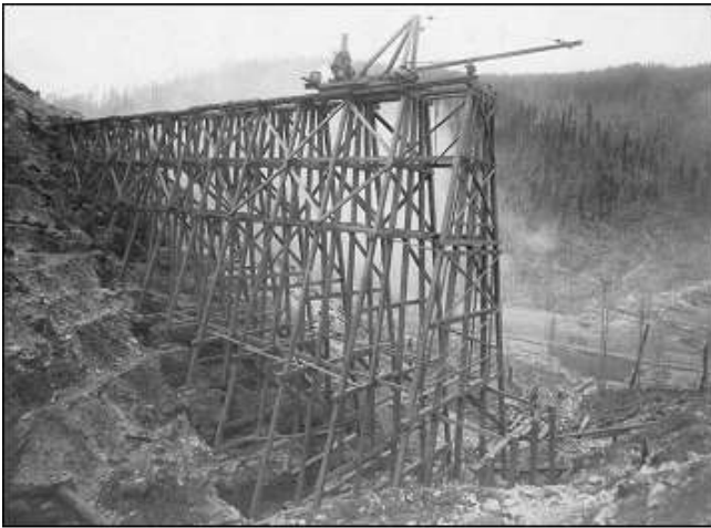
Construction of the fourth trestle on St. Paul Pass.
